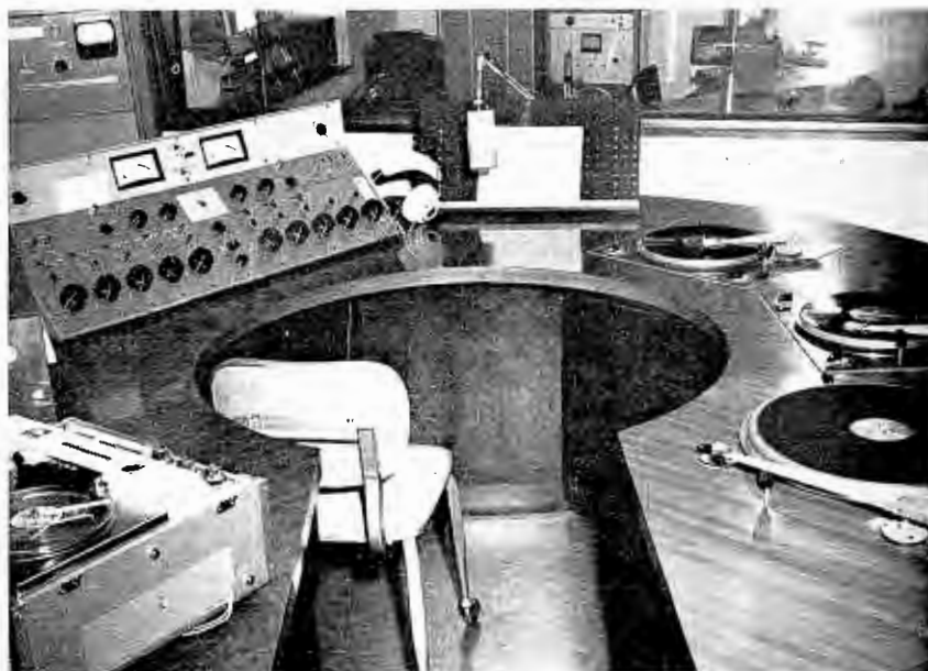
Fig. 2. Completed console desk with all equipment installed.
